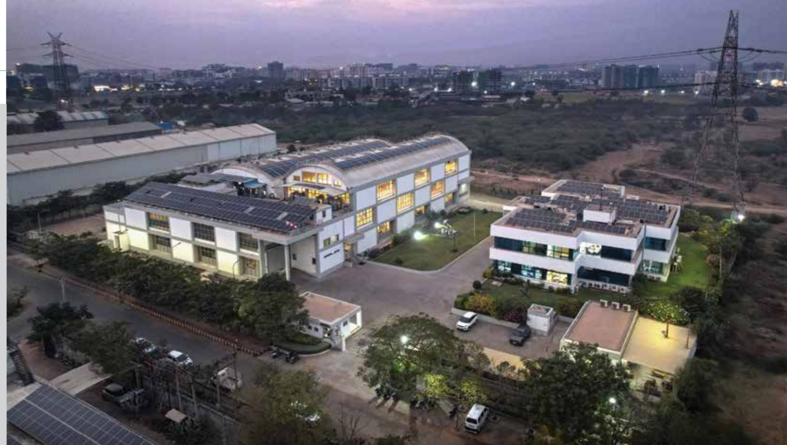
At its Ahmedabad plant, DESMA has established a 350-kW solar energy plant and a water recycling (STP) plant.
