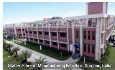
State-of-the-art Manufacturing Facility in Gurgaon, India
